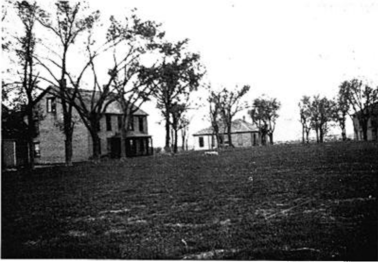
FIG. 23. Old Fort Sisseton, looking across the parade ground to the officers' quarters.
