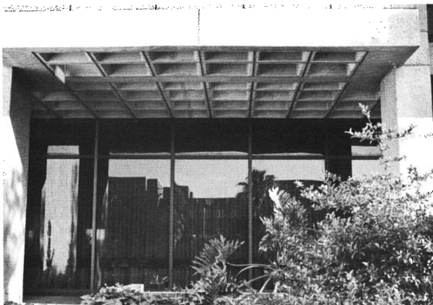
Figure 1. Part of the University of Arizona Main Library showing the exposed section of concrete waffle slab that sheltered the Cliff Swallow nest used by the Cave Swallows. All photos/T. R. Huels.
