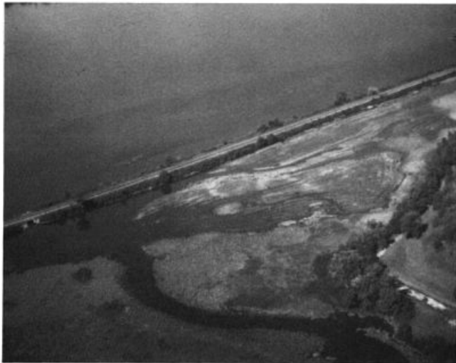
Fig. 2. Aerial photo of Vanderburg Cove showing embayment, railroad causeway, and Hudson River.
