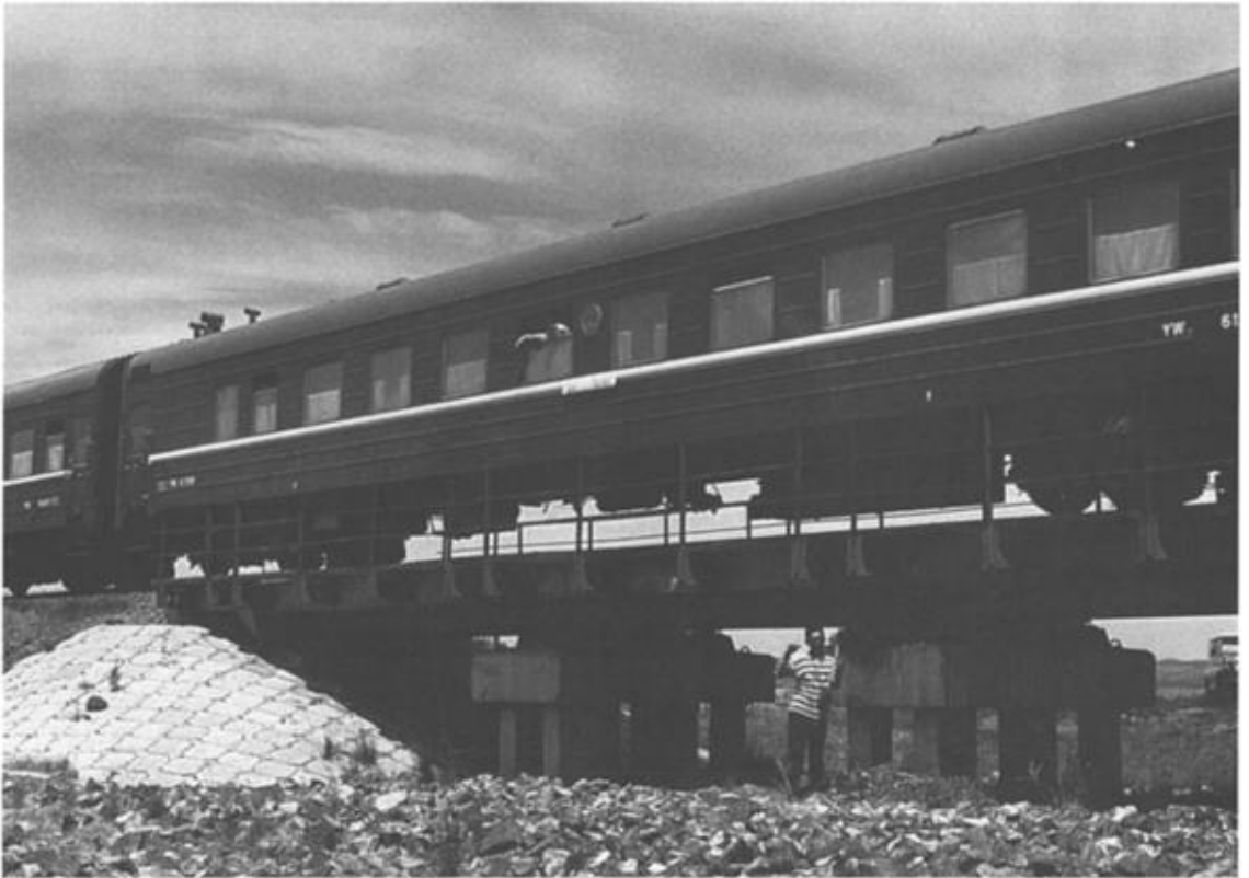
Figure 1. A saker nest 2 m from the ground on an active railroad trestle.
