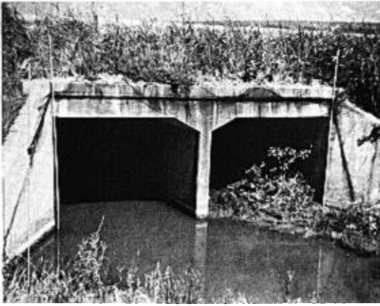
FIGURE 1. Nesting site of Barn Swallows in culverts under heavy-duty road near Madill, Marshall County, Oklahoma. There were 17 active nests in culvert on left and 4 active nests in culvert on right. Note closed mist-nets at entrance of culvert.
