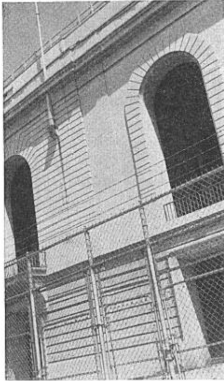
Fig. 32. Feeding area of Black Phoebe on west wall of Memorial Stadium.
