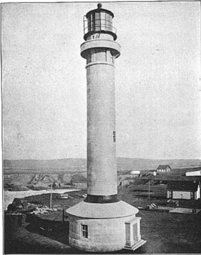
Fig. 2. Lighthouse at Point Arena, Mendocino County, California. The "brick chimney" type, whose great height makes it dangerous to birds. The light at this station is 155 feet above the sea, and the keeper reports from ten to thirty birds per night killed on calm, dark nights during the migration seasons.
