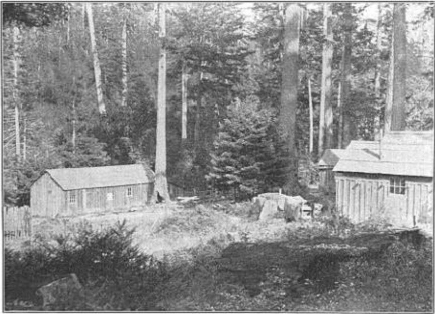
CABINS AT BOVEA CREEK DAM, SANTA CRUZ MOUNTAINS
