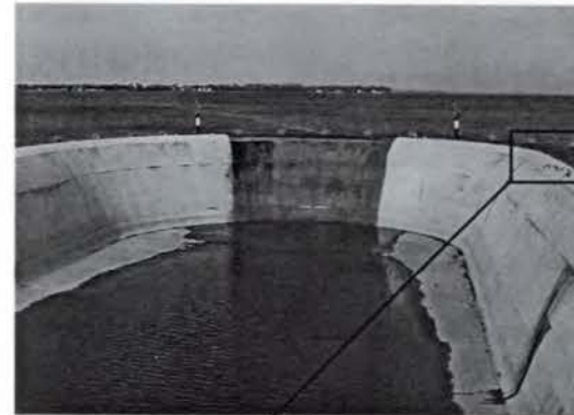
The new spillway at Grand Lake St. Mary's May 1997
