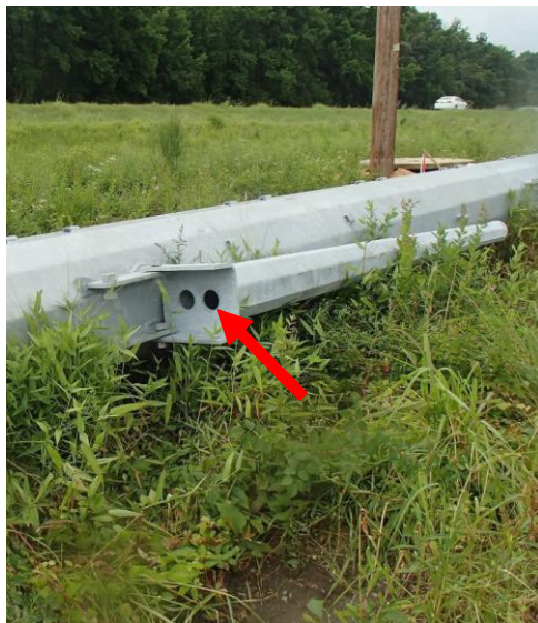
Figure 3. Detail of the 8-cm (3-in) holes providing American Kestrel nesting access to the hollow cross-arm.
