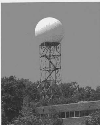
Figure 3: The Boston (BOX) WSR-88D radar in Taunton, MA — photograph by the author
