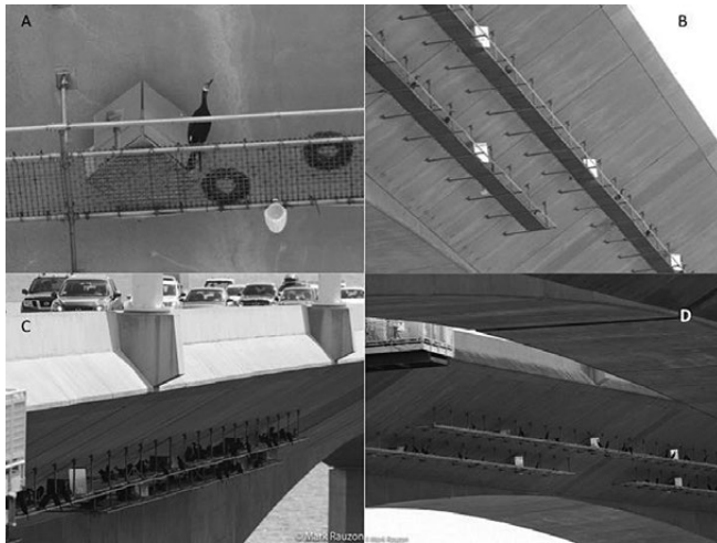
Fig. 3. New San Francisco-Oakland Bay Bridge “Corm Condos” specifically designed in 2001: (A) decoy, mirror box, sound system, and artificial nests made of Christmas wreaths added in 2012; (B) platforms went unused for six years; (C) platform positioning on New Bridge relative to traffic; (D) adoption of platforms after old bridge was demolished in 2017.
