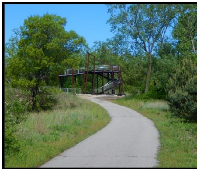
Longshore bird tower at Indiana Dunes State Park as seen on the paved sidewalk approach.
